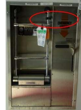
REMOVE CLIPS AT EXISTING EYE WASH
