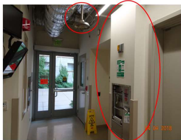
REMOVE EXISTING EYE WASH UNIT AND WALL PROTRUSION
