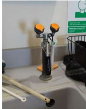
REMOVE EXISTING SINK MOUNTED EYE WASH
