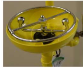
Existing Eye Wash Unit
