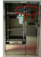
REMOVE CLIPS AT EXISTING EYE WASH
