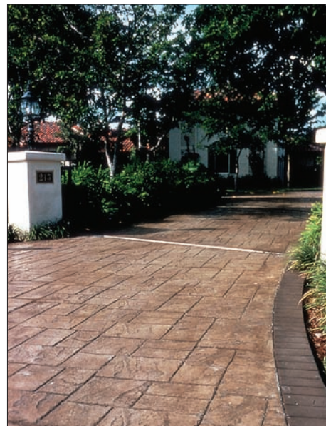
Pattern stamping and colored release agents are applied to integrally colored concrete for unique effects.
